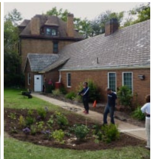
Rain garden installation at the Biddle Bldg.
