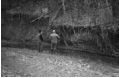
Examining an unstable stream bank
