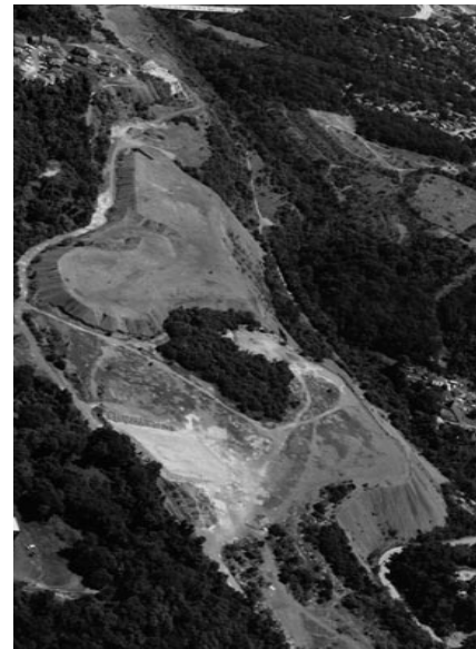
An aerial view of the slag dump looking towards I-376.
